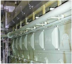
SELCO offers a versatile range of control and monitoring units for diesel and gas engines. The range includes start/stop control units with built-in monitoring of critical engine para-meters, as well as separate emergency shut-down units.
