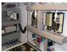
The M0200 continuously reads engine speed, oil pressure and cooling water temperature from the ECM of the the M2000 from the discreet contact outputs. The M0200 supports the cable check function of the M2000.
