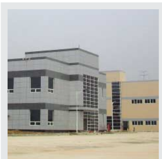
Wuxi Plant (China)
