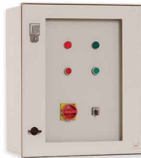
Using internal door with a transparent window is a good solution for the fixing of signal and measurement elements.
